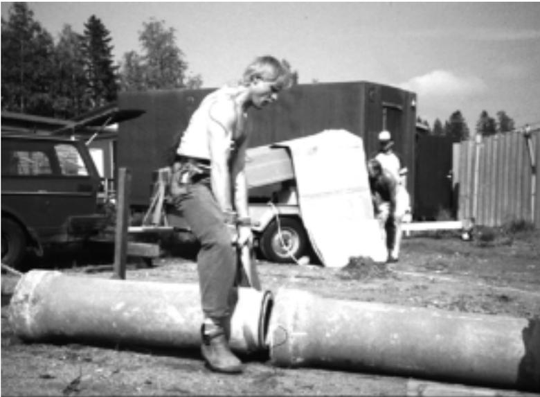
Figure 8. Fitting drain pipes with the new method.
