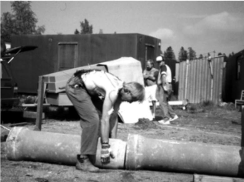
**Figure 7. Fitting drain pipes with the old method.**
