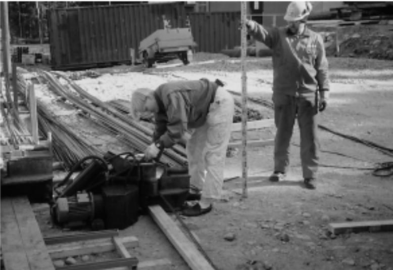
**Figure 3. Moving and cutting concrete reinforcement rods with the old method.**
