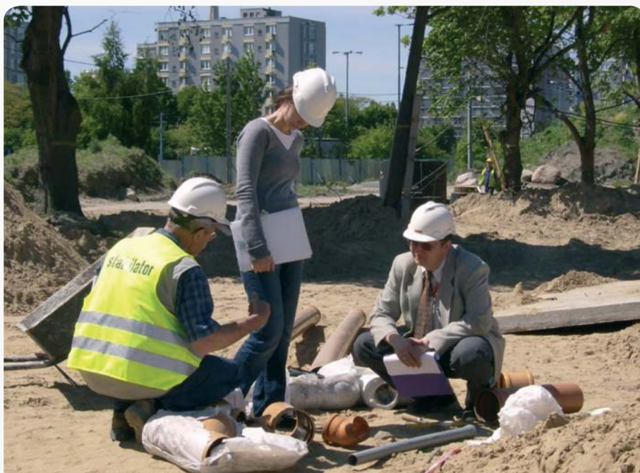
Fot. Stabilator Sp. z o.o.
